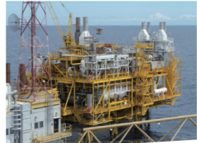
Offshore gas treatment plant
